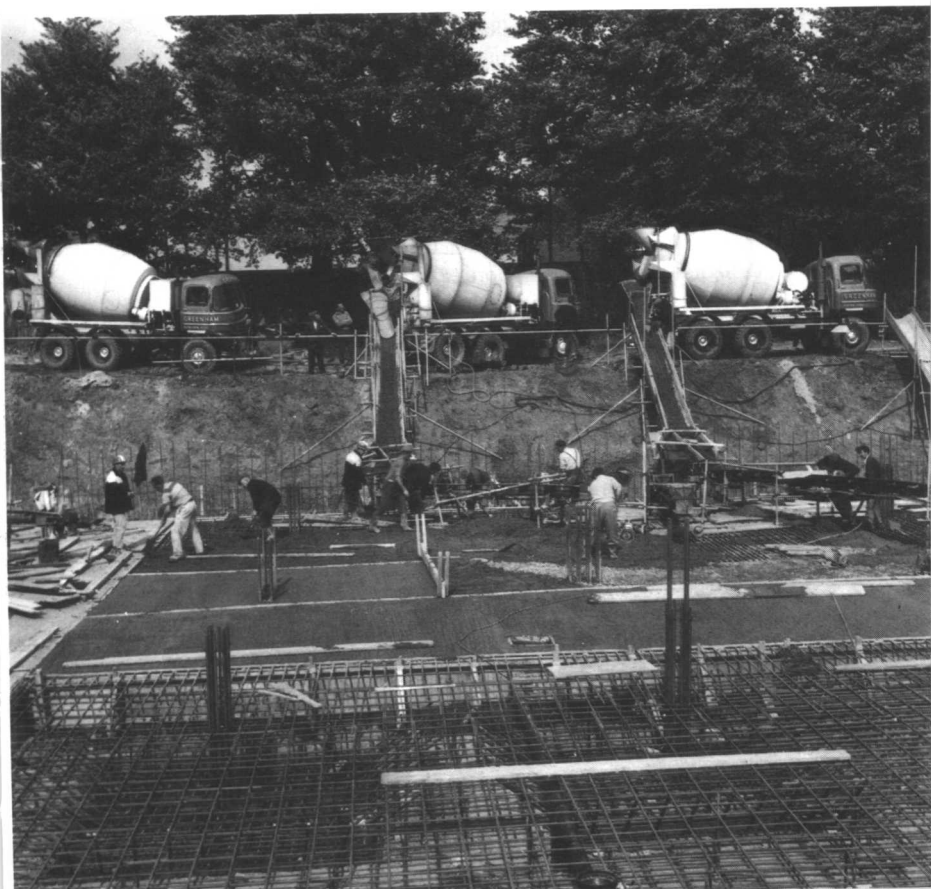
Lorries delivering ready-mixed concrete
