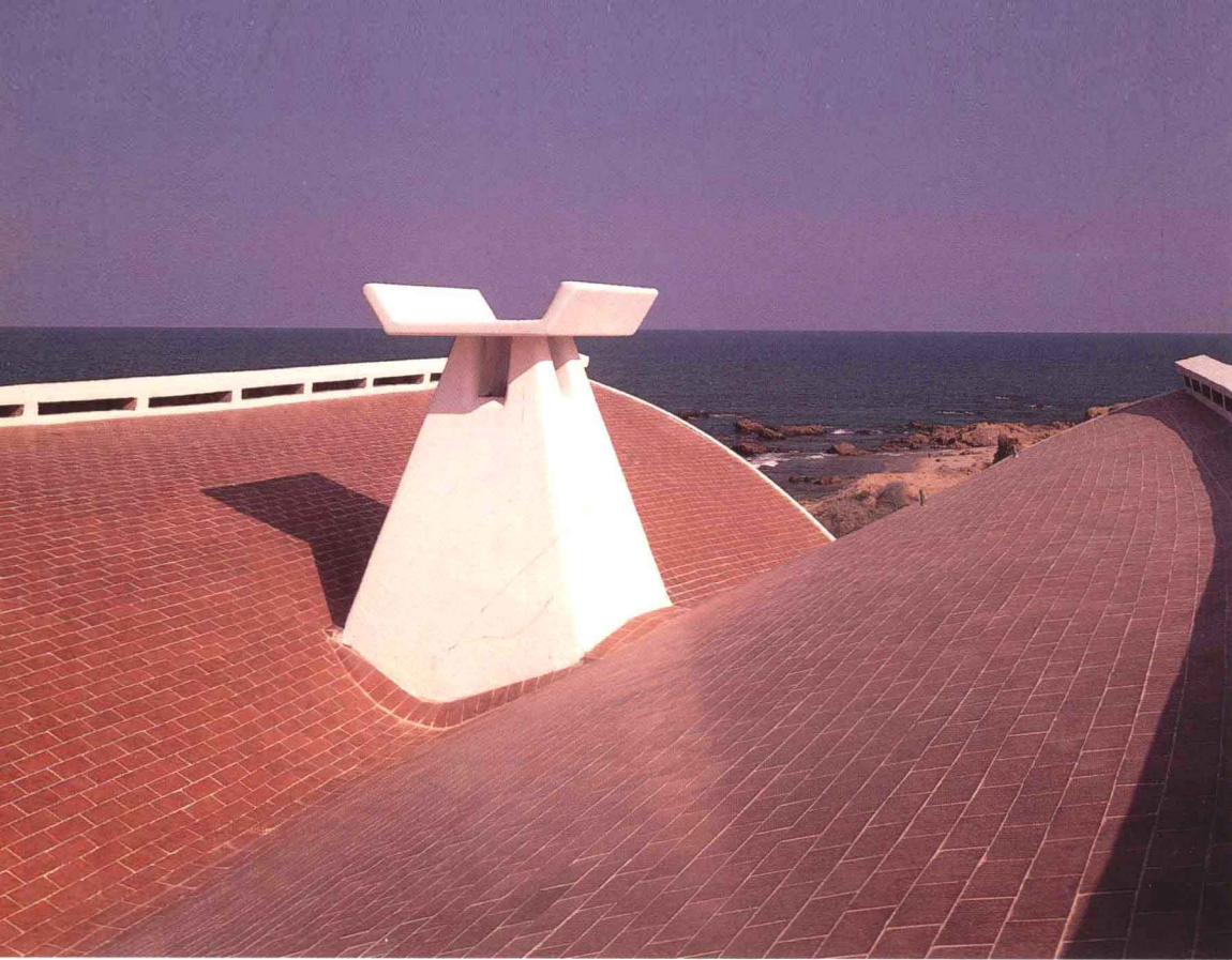
LEFT: Detail of the tile roof, with venting in center and at edges. This roof's structure is composed of lenticular trusses, which give it its unique shape. Photo: Alan Weintraub, funding by the Graham Foundation.
