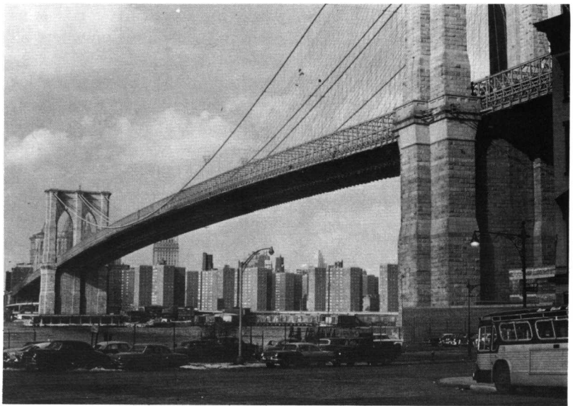
Figure 1.1 Brooklyn Bridge across the East River in New York
