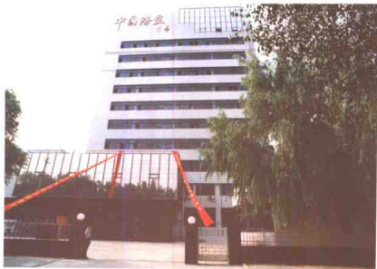
秦皇岛海监局办公大楼 The building of MSA of Qinhuangdao
