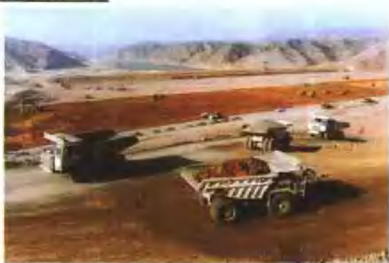
拦河大坝填筑
