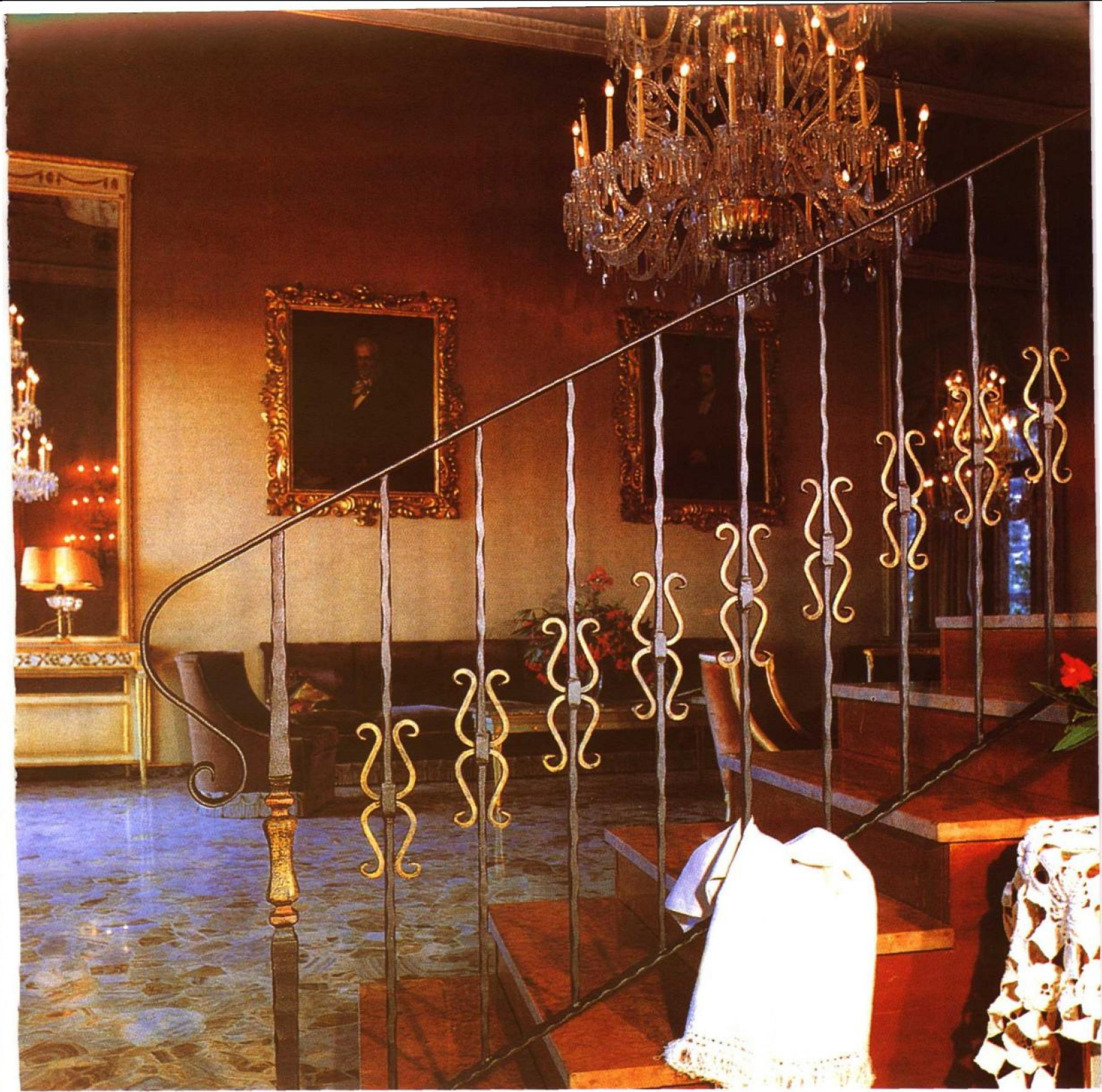
铁艺锻件基本单元: 900 × 150mm, 20 × 20mm
