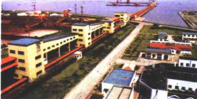
上海罗泾煤码头成套装卸设备和控制系统。 Loading/unloading Equipment and Control system.
