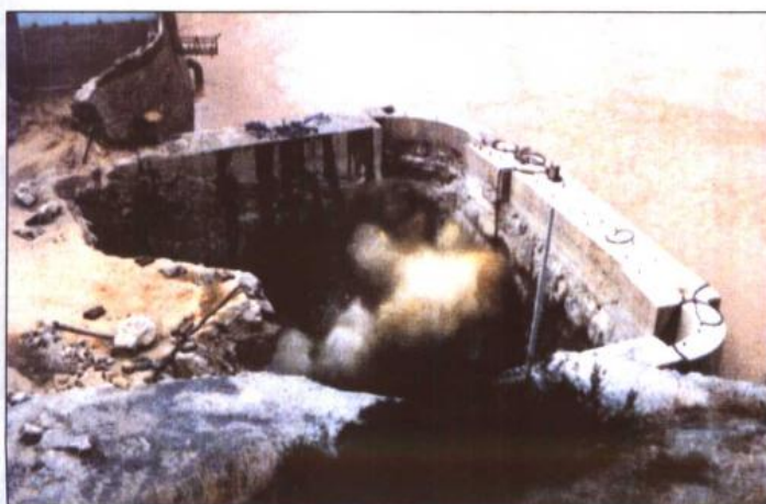
7-2 泵站基坑开挖
