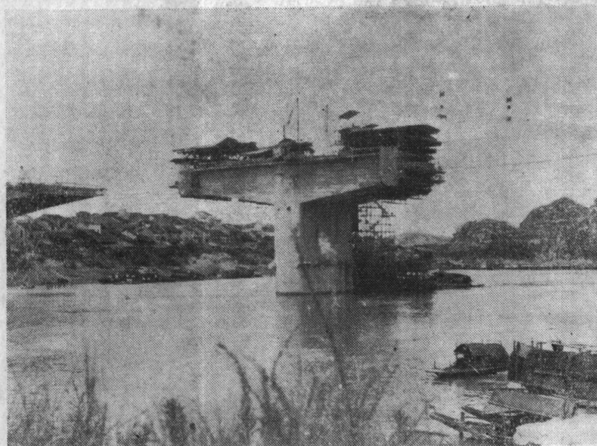
节段顶板钢索张拉
