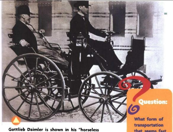
Gottlieb Daimler is shown in his "horseless carriage" in 1885. His son, Wilhelm Daimler, is in the driver's seat. The car was a converted horse-drawn wagon with a gasoline motor.
