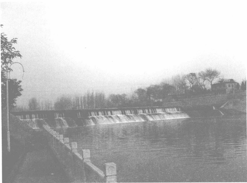
禹州颍水橡胶大坝
