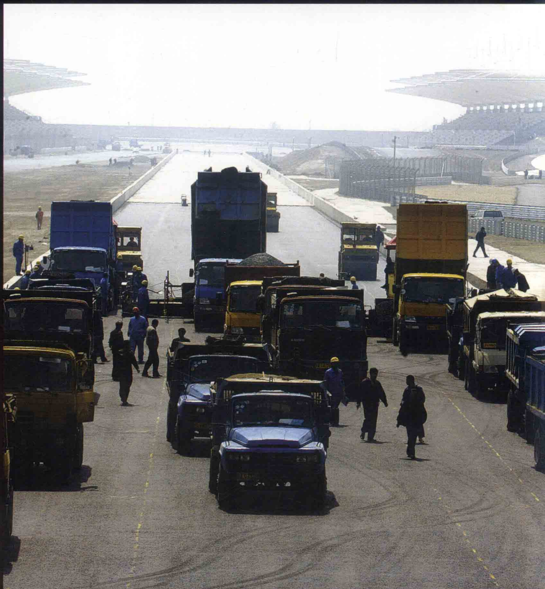
赛道沥青层摊铺 The asphalt layer of the racing field is in pavage.
