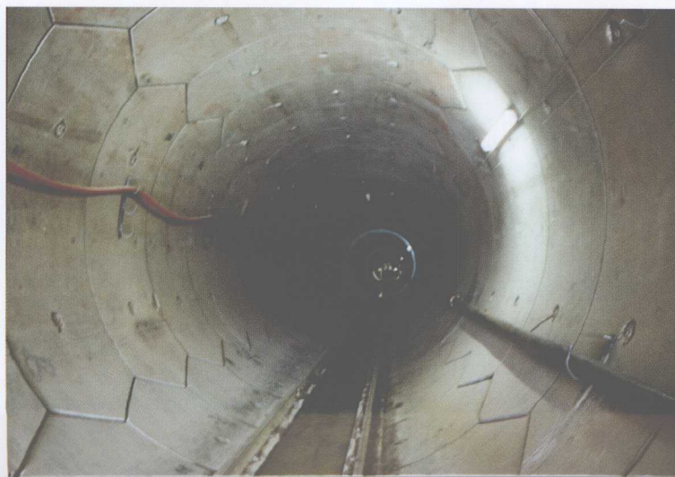
TBM成洞
