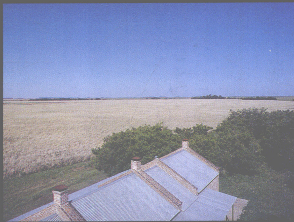
This Page: House in San Martin roof (top), House in El Salado (bottom left), and House in El Talar (bottom right).
