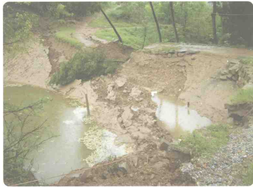
池塘被毁, 池水入渗促使滑动加剧 Sliding destroyed this pond; then water seepage worsened sliding
