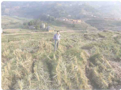
稻田水渗入滑坡体, 促进了滑坡的变形拉裂 Water seepage from rice field increased deformation and cracks
