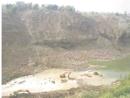
滑坡剪出滑入江, 形成滑坡坝体 The sliding mass fell into and dammed the river
