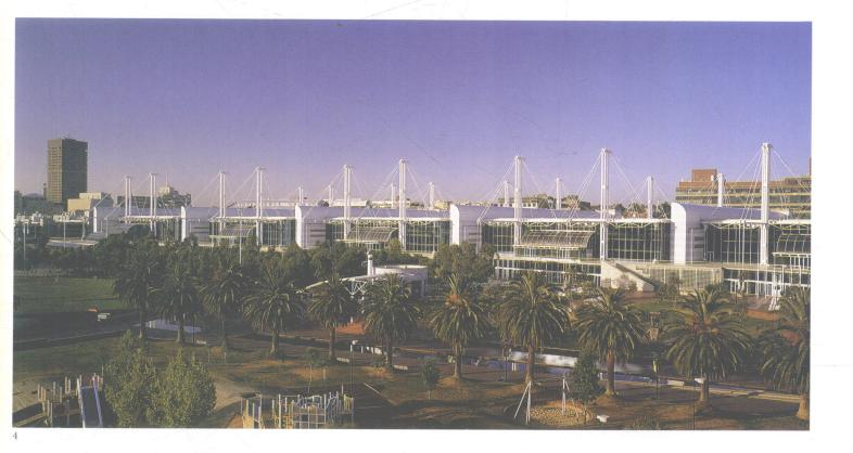
These objectives were met by a continuous mast and cable structure, proving to be economical and also allowing a low horizontal scale to be developed.
