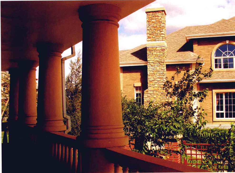
↑ 别墅内侧走廊的眺台 The view platform of insider corridor
