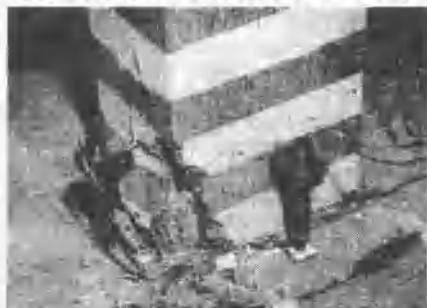
Fig. 8 Damage at Column Base
