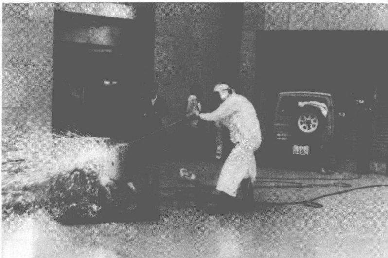
Figure 6 Thermal lance set-up and operation (Courtesy of Hong Kong Oxygen & Acetylene Co. Ltd.)
