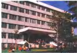
第一教学楼(北院) No.1 teaching building
