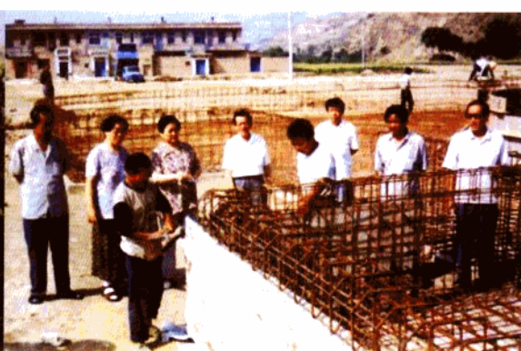
△县政协领导视察积翠公园施工现场
