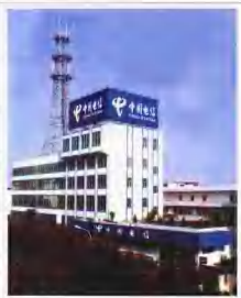
电信大楼 Telecommunications Building
