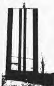
FIG. 1 MCKINLEY BUILDING: EARTHQUAKE DAMAGE IN NORTH END WALL
