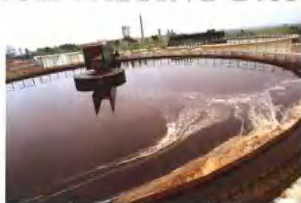
污水处理厂 Sewage treatment plant
