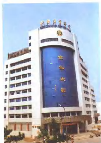
农业银行昌邑支行大楼 Agricultural Bank Changyi branch building
