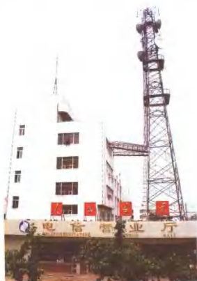
电信大楼 Telecom building
