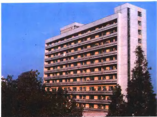
病房大楼 The in-patient building
