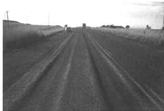
Figure 5 A Unique Manifestation of "Accelerated" Pavement Distress due to Traffic on a Regional Road R103 (formerly N3) near Warden, South Africa.
