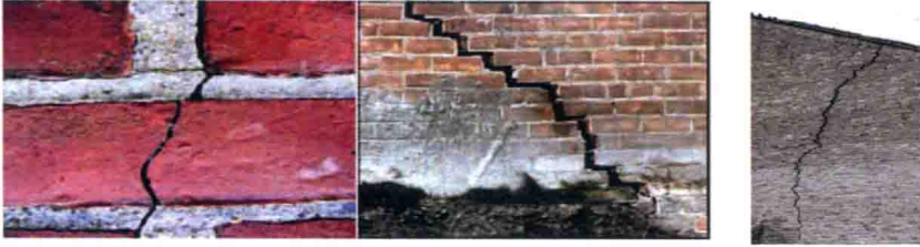
Figure 1. Fracture of detachment in brick walls at different scales
