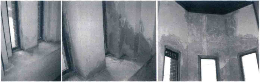
Figure 2: Observed moisture damage in the tower of the building: moist spots and efflorescence.
