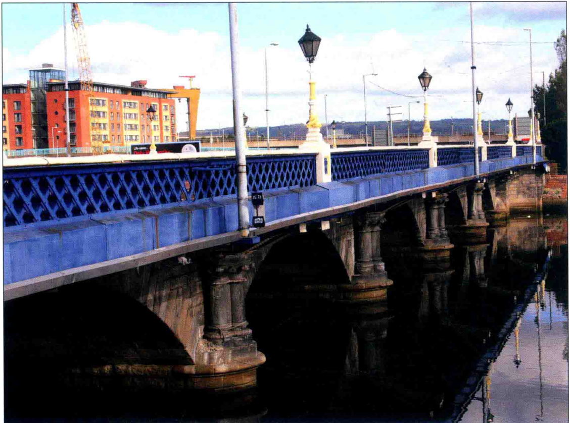
Queen's Bridge, Belfast, showing its original 1844 stone arches and its later cantilevered iron extensions. (Ardfern: Reproduced under the Creative Commons Attribution-Share Alike 3.0 Unported license)
