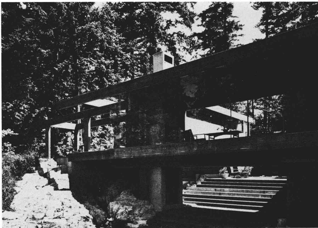
The beams and columns supporting the Smith House are of the same width and section and similar in size and scale to the surrounding trees.
