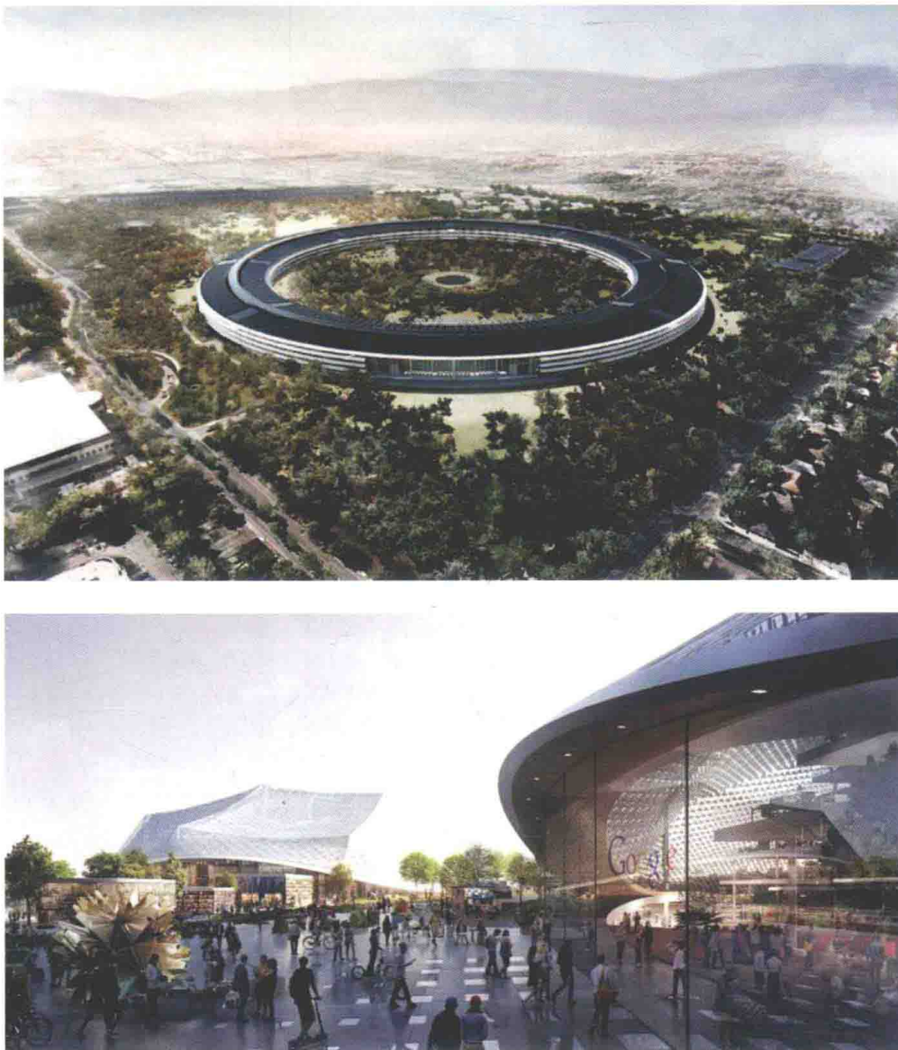
Figure 1.1 Apple Campus 2 is an NZE building designed to generate all the energy it requires from photovoltaic (PV) panels located on its circular roof. Its many passive design features allow it to take advantage of the favorable local climate such that cooling will be required just 25 percent of the year. (Source: City of Cupertino, September 2013)
