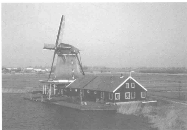
Figure I.1 Restored 18th-century Dutch windmill used for grinding grains. Others were used for pumping water.
