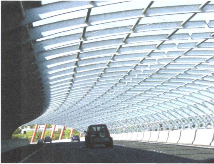
The sound tube in Melbourne, Australia is designed to reduce roadway noise without detracting from the area's aesthetics
