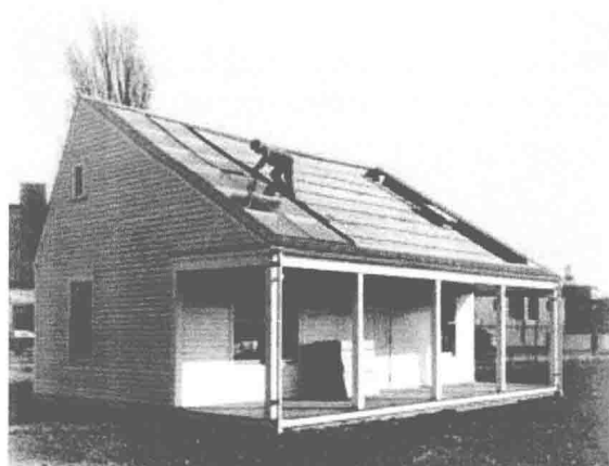
MIT's Solar House #1, built in 1939 in the U.S., used seasonal thermal energy storage for year-round heating.
