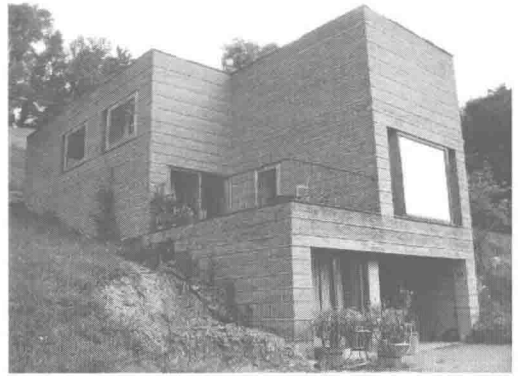
Figure 6. Rauch House: 3 storey loadbearing unstabilised RE.
