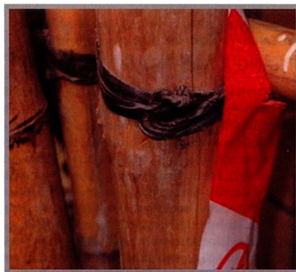
FIGURE 2 Lashings that secured the bamboo poles of the Hong Kong scaffolding had no knots. They were secured by turning back on themselves and wrapping in a knotless manner.
