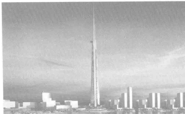
Fig. 1.6 Proposed 1 km high tower in Jeddah, Saudi Arabia; it will require half million cu.m of concrete
