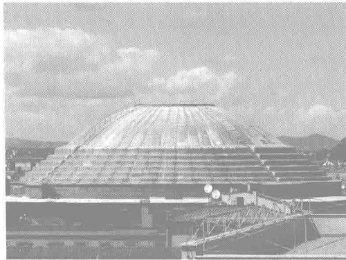
Fig. 1.1 Ancient roman pantheons (Temple of Gods); built in 128 AD, it has 43.2 m diameter dome, a record for 1800 years
