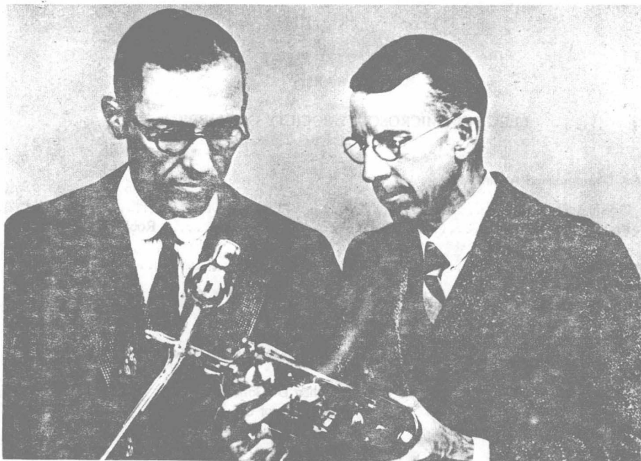
In 1927, Clinton J. Davisson (right) and his associate, Lester H. Germer, with the tube they used in their classic experiments.
