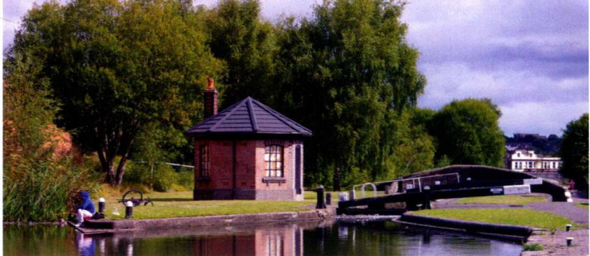
Smethwick Lock, formerly duplicated. The chamber on the left side has been filled in.
