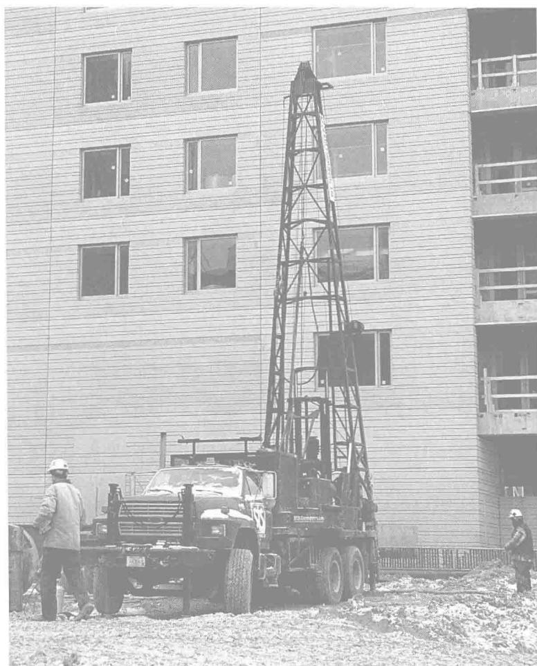
Figure 1-3. A geotechnical investigation rig. The investigation is usually performed before the contractor is hired, as part of owner due diligence, and the results are published in a geotechnical or soils report, which could be part of the bidding documents. Soil samples can be extracted in driven sampler tubes for analysis. The results are displayed by boring logs, which commonly give the soil classifications, soil moisture contents, and penetration test blow counts at various depths. The log also shows the groundwater level, which might fluctuate over time to affect construction operations.
