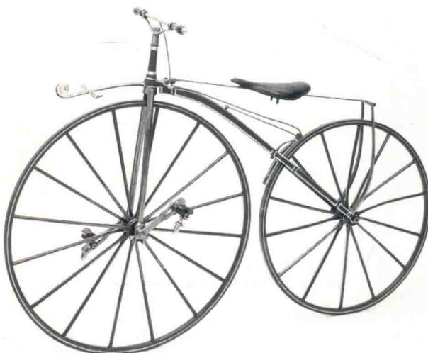
Figure 1-1 The motorcycle is a direct descendant of the early bicycle, which was actually called a velocipede because of the placement of the pedals on the front wheel.
