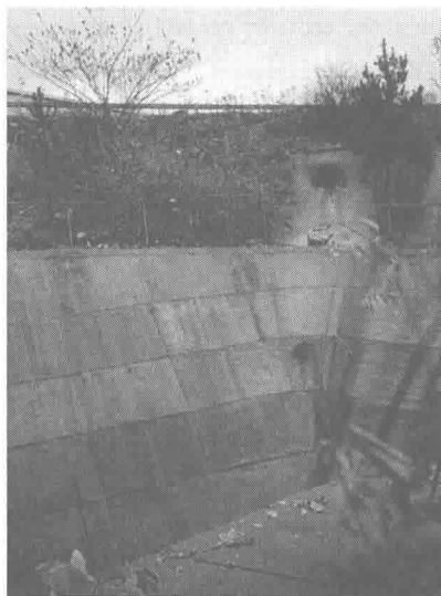
Figure 2. Dry Detention Basin, Culvert and Rundown with Safety Concerns Due to Steep Side Slopes and No Egress or Escape Route
