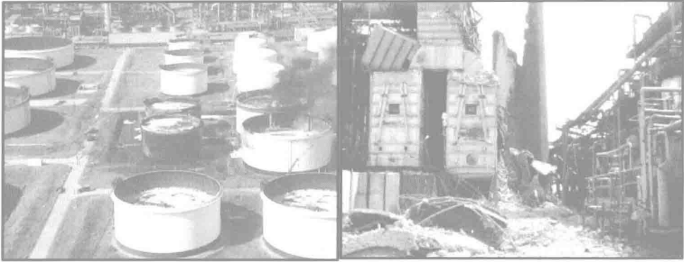
Figure 1: Damaged tanks at tank farm (left) and collapsed stack at TÜPRAS Refinery
