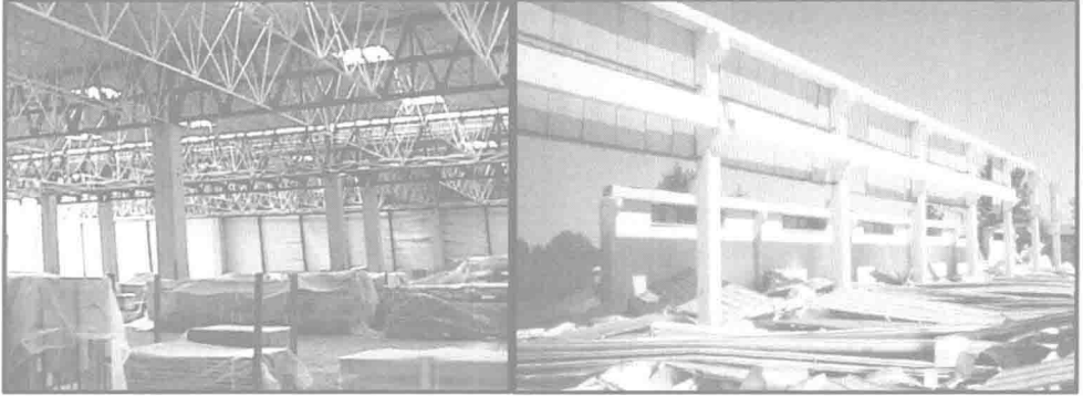
Figure 3: Damaged prefabricated buildings at Ford Otosan Plant
