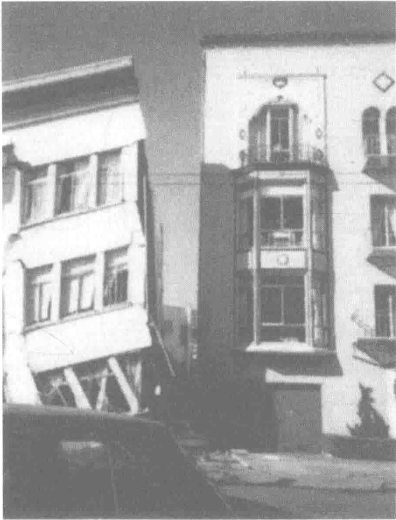
Fig. 1.2 Collapse of a building (Loma Prieta earthquake, 1989) (reprinted from Kasai and Maison 1997 with permission from Elsevier)
