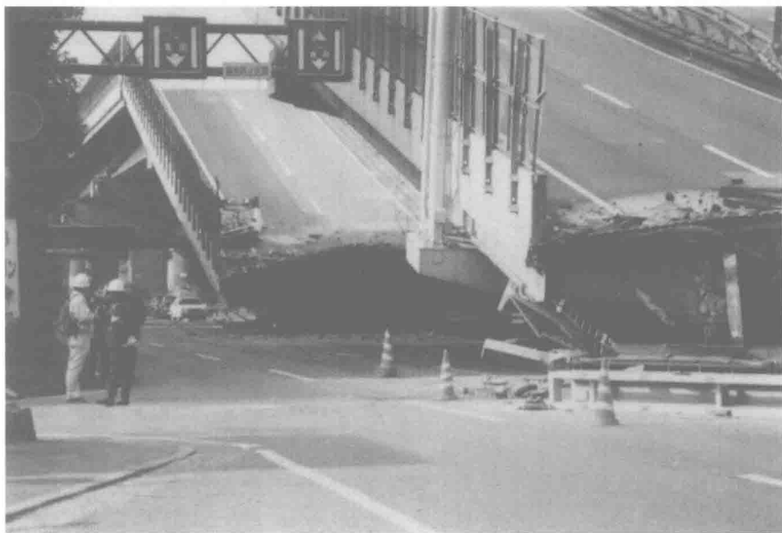
Fig. 1.4 Pounding as one of the reasons for falling down of superstructure segments (Kobe earthquake, 1995)
