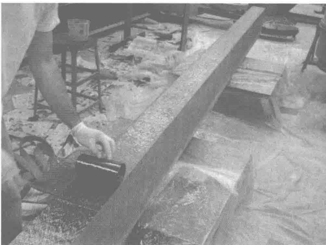
FIGURE 1.1 Strengthening the soffit of inverted reinforced concrete beam with CFRP.
