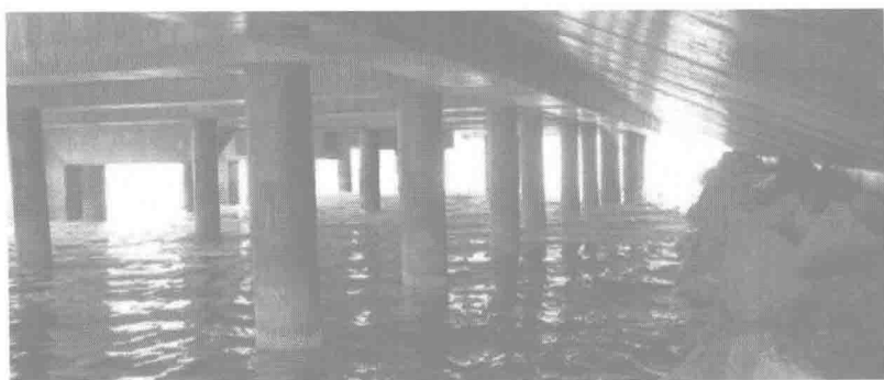
Figure 1.2 Open concrete structures are still the most common type of harbor structures built along the Norwegian coastline.
