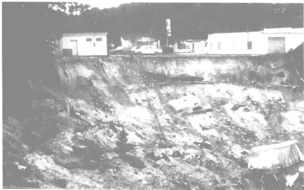
Figure 3 Sinkhole occurrence in area underlain by carbonaceous (limestone family) rock. (Source: USGS photo)
