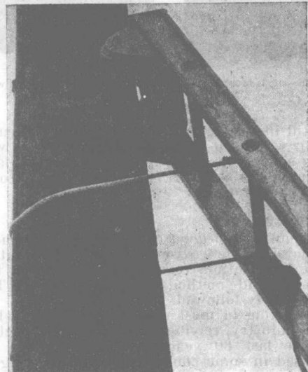
FIG. 343. A proprietary captive device for lashing the head of a linesman's ladder to a telegraph pole. (By courtesy of the Postmaster-General, United Kingdom.)
