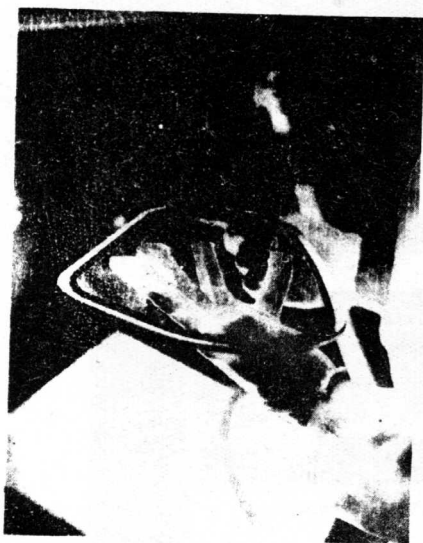
Fig. 7 Adhesively joined window for Apollo spacecraft. ( North American Aviation. )
