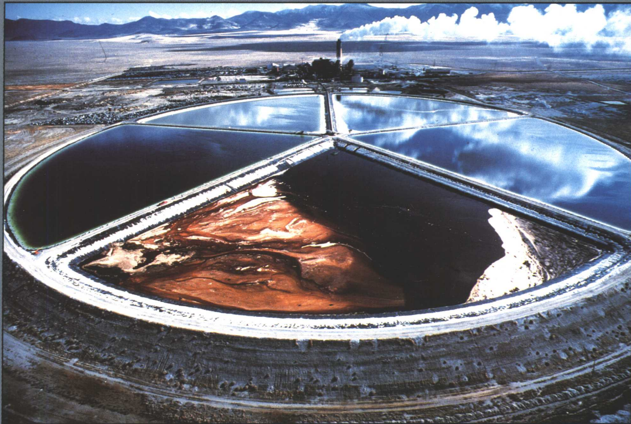
Magnesium bromide and magnesium chloride are obtained by solar evaporation of salt water.
